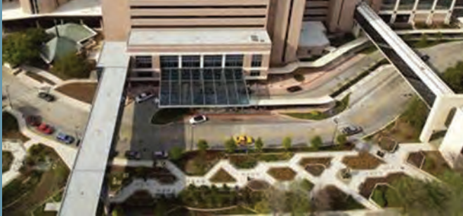
Figure 26: This aerial view of Texas Medical Center illustrates the creation of landscape buffers to enhance stormwater management.
