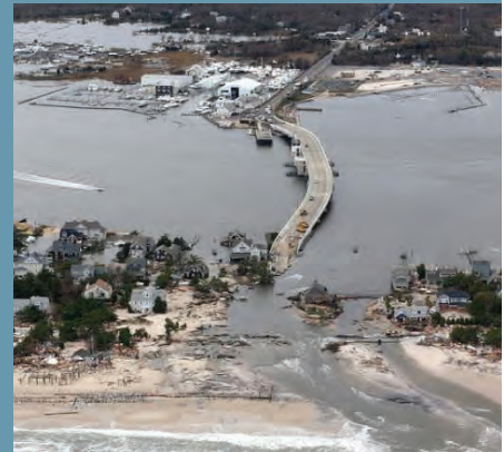
Figure 23: This washed out bridge along the New Jersey shore following Superstorm Sandy demonstrates how vulnerable residential shoreline communities can become disconnected from transportation infrastructure; if large numbers of medical personnel live in such communities, hospitals and long term care facilities must plan to relocate those staff prior to major storm events.
