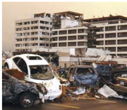
Figure 22: Debris outside the Joplin Hospital Emergency Department, following the EF-5 tornado, complicated evacuation procedures.
