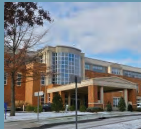
Figure 18: The Greenwich Hospital's on-site combined heat and power system operated without incident throughout the 7-day loss of utility services following Superstorm Sandy.
