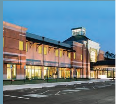
Figure 15: Louisiana Heart Hospital, designed to withstand high winds, successfully operated through Hurricane Katrina
