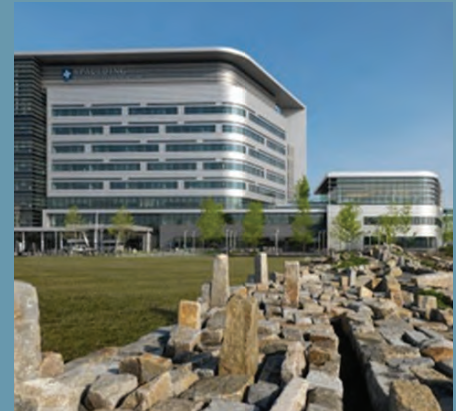
Figure 11: Spaulding Rehabilitation Hospital, completed in 2013 on the Boston waterfront, includes such resilience features as an elevated first floor and roof-mounted electromechanical infrastructure.
