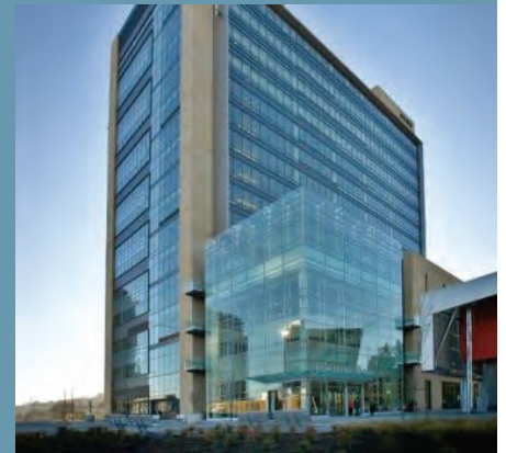
Figure 20: The Oregon Health and Sciences University Center for Health and Healing uses four separate water systems to reduce reliance on both the municipal potable water system and sewage treatment system. It captures, treats, and recycles the building sewage conveyance water using an on-site bio-reactor system.
