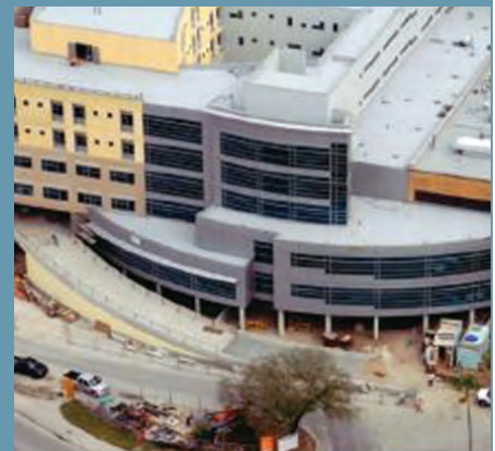
Figure 21: Tampa General Hospital's emergency department is on the second floor, well above the flood surge and inundation level. The vehicular ramp is shown here.
