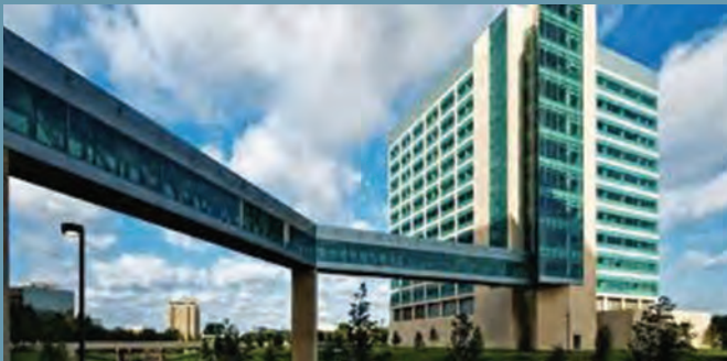
Figure 28: Texas Medical Center improvements include elevated walkways that provide utility distribution as well as advanced stormwater management strategies.
