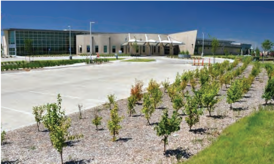
Figure 25: These bioswales at Kiowa County Memorial Hospital filter stormwater and support the Ogallala Aquifer recharge. Rooftop rainwater is collected for irrigation and toilet flushing.
