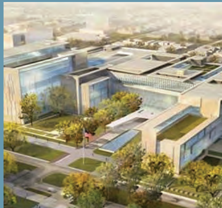
Figure 24: The new Southeast Louisiana Veterans Health Care Center (SLVHCS) features a range of enhanced resilience and infrastructure planning measures. The building is designed to operate for a minimum of seven days, even if all of New Orleans’s utility and infrastructure services are lost.
