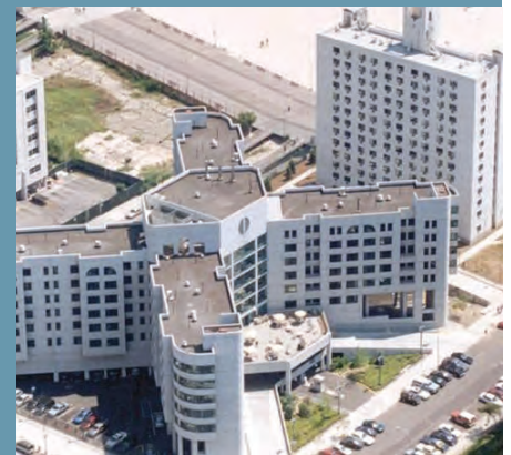
Figure 14: Shorefront Rehabilitation Center, Brooklyn, NY, functioned as planned during and after Superstorm Sandy. The structure was designed to accommodate storm surge at its base levels; all critical infrastructure is above flood elevations.
