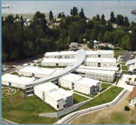
Figure 17: Washington State Veterans' Home orients resident wings to maximize passive cooling and prevailing winds, and includes engineered natural ventilation to replace air conditioning.
